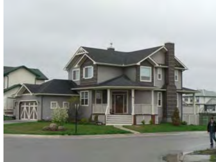
An example of a chimney.
