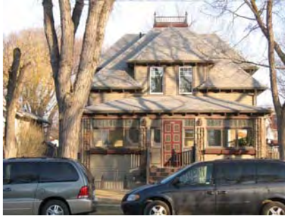
An example of a widow's walk and soffit brackets.
